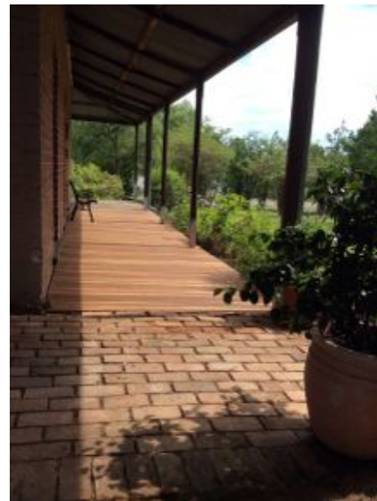
The new floor of the verandah
